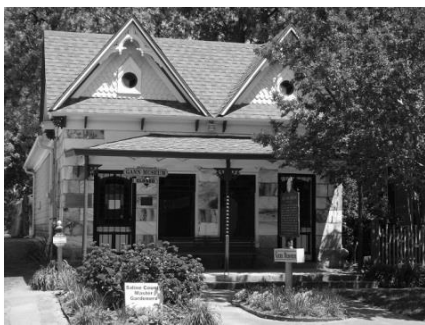
Gann Building, Benton, Saline County
