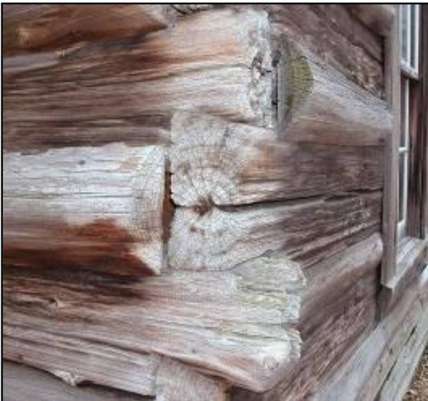
**5. Cracks between the logs were filled in.**
