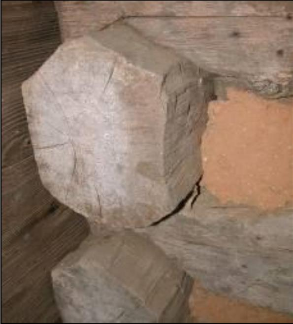
**4. The ends of the logs were dovetailed (4 corner notched) to let the rain slide off the end of the log, so the wood wouldn't decay.**
