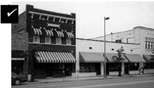
The primary entrances to buildings are recessed, providing a shaded area that helps to define doorways and to provide shelter to pedestrians. This feature should be repeated on new infill buildings along Main Street.
