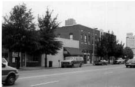
Uniform facade widths evenly spaced along Main Street create a rhythm that contributes to the visual continuity of the area.
