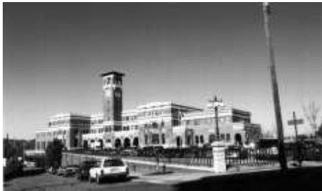
The Union Station neighborhood should develop with a mix of uses that supports the adaptive reuse of the station itself.
