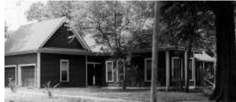
An addition should be compatible in form, scale and materials with the historic building. Using a "connector" to link the new construction with the original is one means of maintaining the character of the primary structure.
