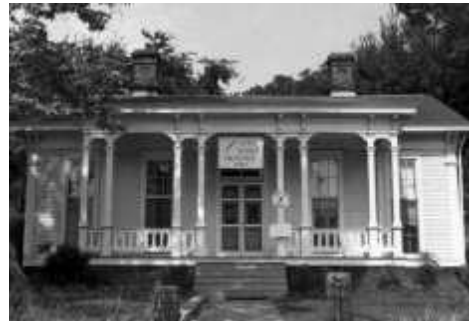
The Old Hotze House is one of the few houses in the Mansion Area with Italianate features. (Photo: ca. 1960)
