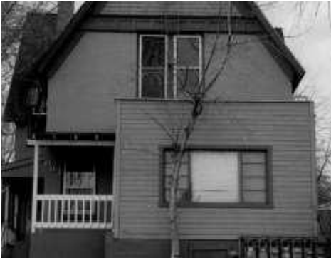
Do not construct a new addition that will hinder one's ability to interpret the historic character of the building or structure. This addition obscures the front porch, for example, and is inappropriate.
