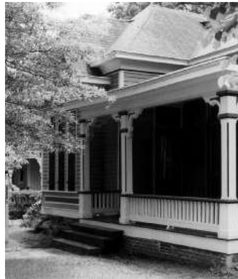
Character-defining features of a porch should be preserved. These include balustrades, columns, brackets and steps, as well as foundations and flooring materials.
