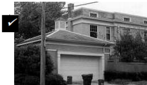
This new secondary structure is a contemporary interpretation of the traditional building and is compatible with the historic context.
