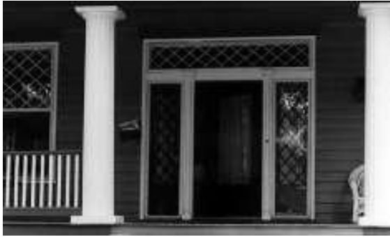
The character-defining features of historic front doors should be preserved.
