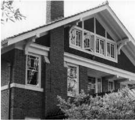
Window frames, brackets, molding and strapwork are examples of architectural features that contribute to the historic significance of a property which should be preserved.
