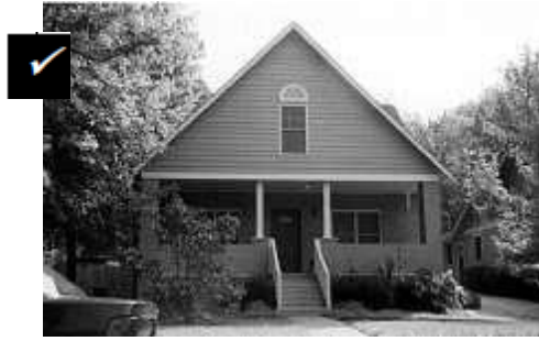
This new infill building appears similar in mass and scale to single-family residences seen traditionally.
