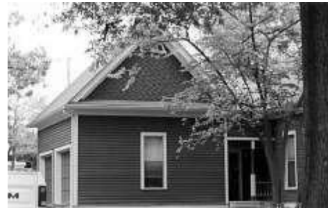
A new porch serves as the connector in the photo above, linking the new construction with the original.
