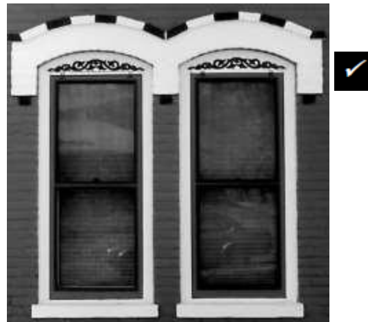
If a storm window is to be installed on the exterior, match the sash design of the original window (as this one does).
